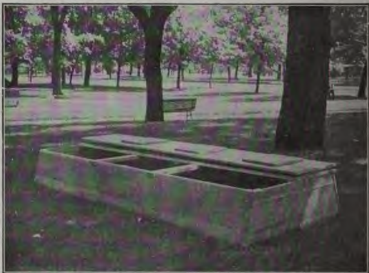
FIG. 212.—The Havard knock-down box, with one-half of the top shifted over the other half for inspection and disinfection.
